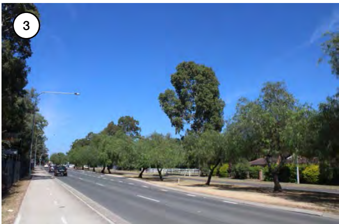
View along Mulgoa Road looking south
